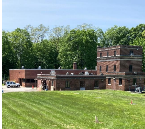
The West Lake Water Treatment Plant produces approximately 4 million gallons of water per day.
