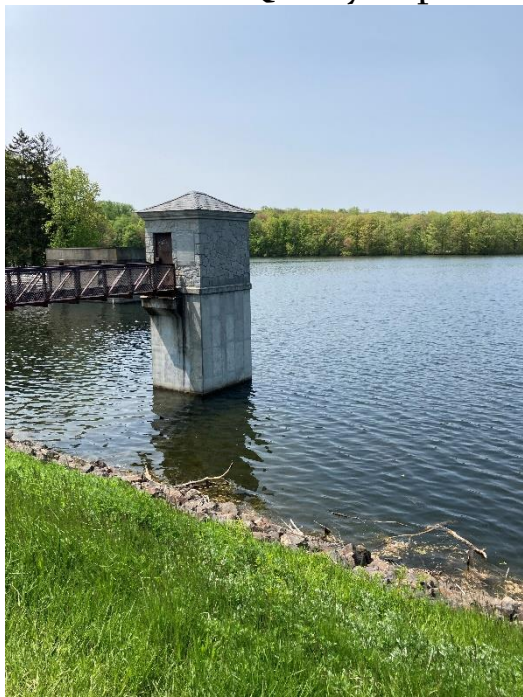
West Lake Reservoir – “old” intake structure
